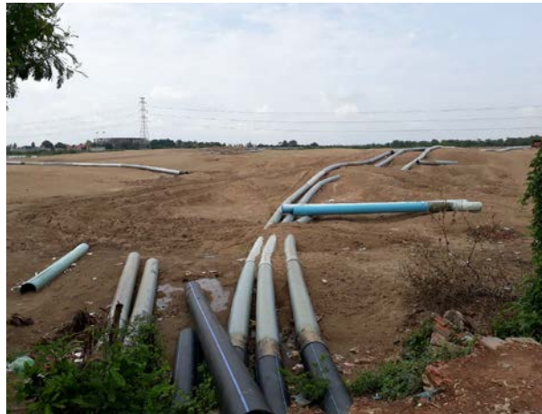
Figure 4. Filling in vast wetland areas like Tompun Lake can take years. Pipes are laid across many kilometres, allowing sand to be continuously fed into the wetland area.
