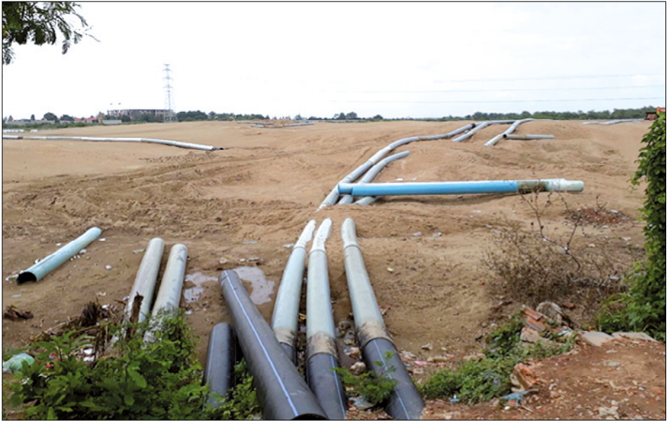
Photo 6. Filling in vast wetland areas like Tompun Lake can take years. Pipes are laid across many kilometres, allowing sand to be continuously fed into the wetland area Credit: L. Beckwith, June, 2018.
