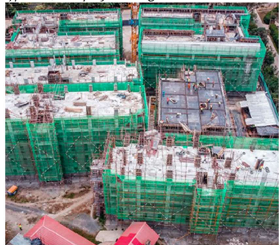
Typical Qwetu project using EPS on slabs
